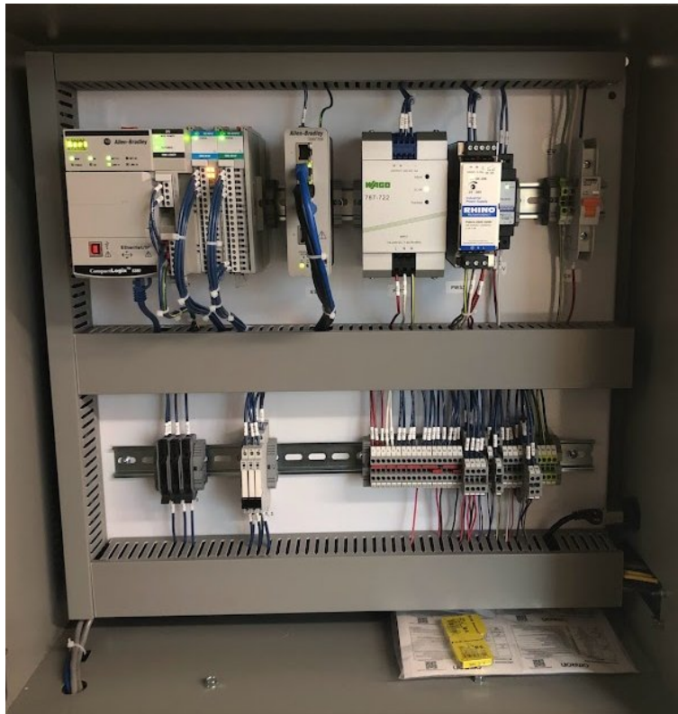
Figure 21: Final Wiring of Control Panel
